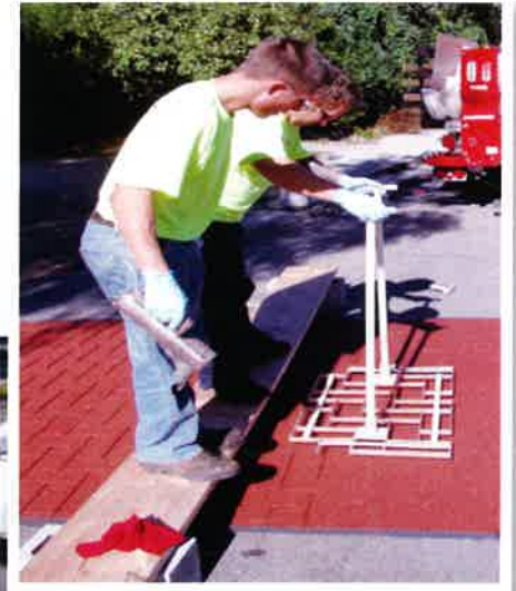
STEP# 5 Mixture is printed
