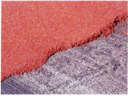
STEP# 4 Mixture luted & troweled to 5/8"
