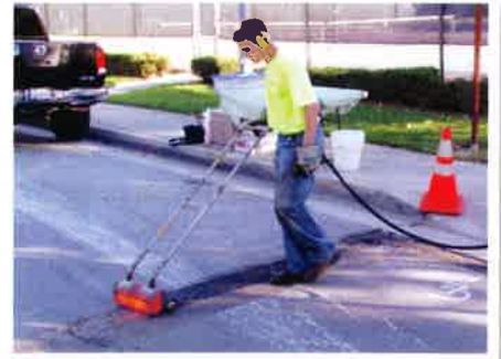
STEP# 3 Hot Compressed air cleaning
