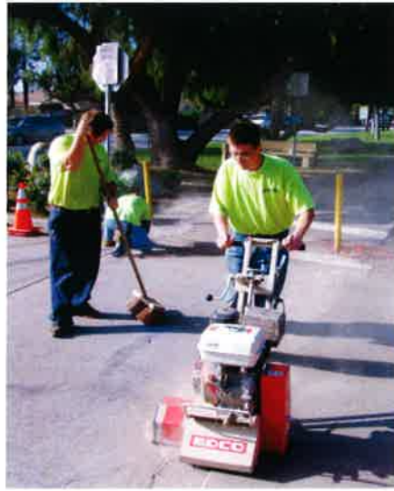
STEP# 2 Grinding 12" wide notch
